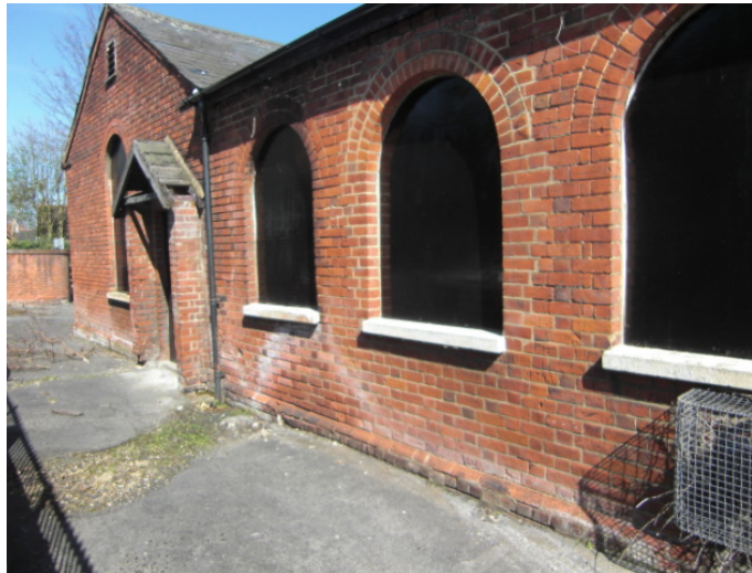
The dilapidated Cowbridge School building
